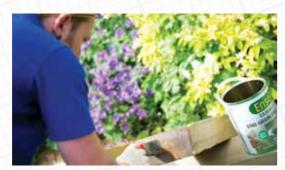
If you need to cut your sleepers to a different length ensure you treat cut ends with endseal preservative. Sleepers are hard work to cut with a handsaw – ask your local timber merchant if they can cross cut to length for you. WARNING: Never use a chainsaw unless you are properly qualified.
